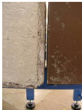
Figure 1-44. Gap between Scattering Box Concrete Blocks.
